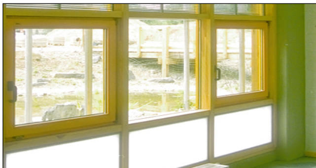
Transparent insulation material in the bottom section of a window assembly.
